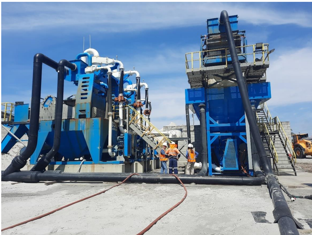
Plate 8 – Primary wash-screen process on right and dewatering units on left
