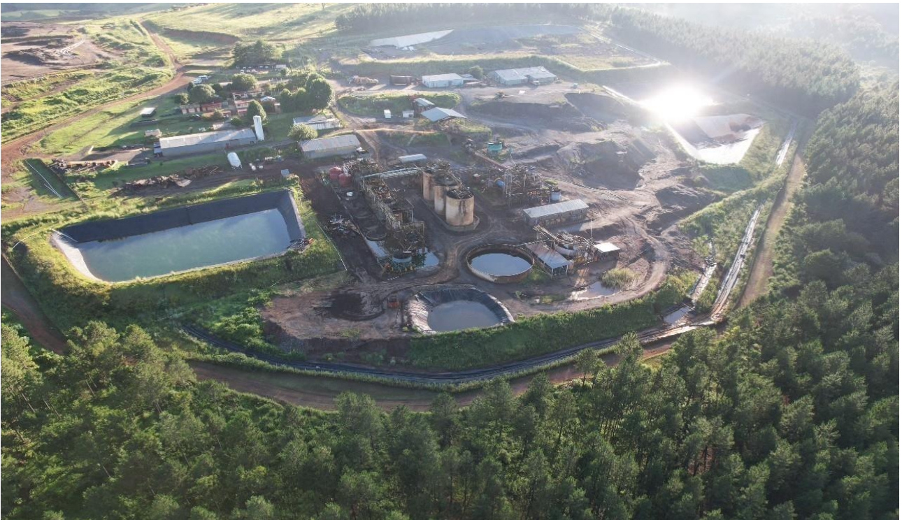
Figure 6: Existing Plant Drone View (post demolition of old sections)
