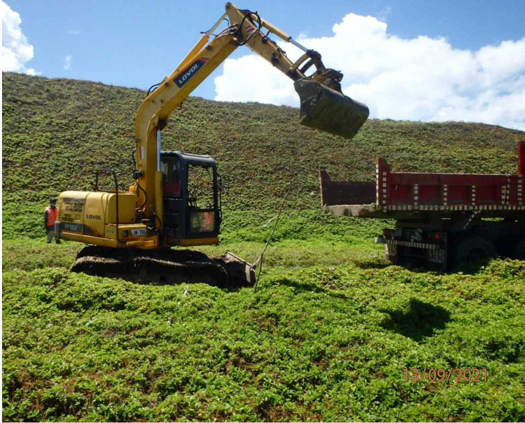
Plate 1 – Excavator and truck on site for bulk sample collection
