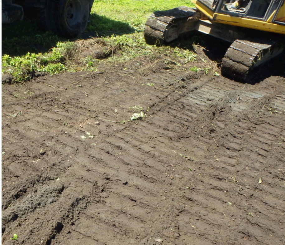
Plate 5 – Sampling site reclamation
