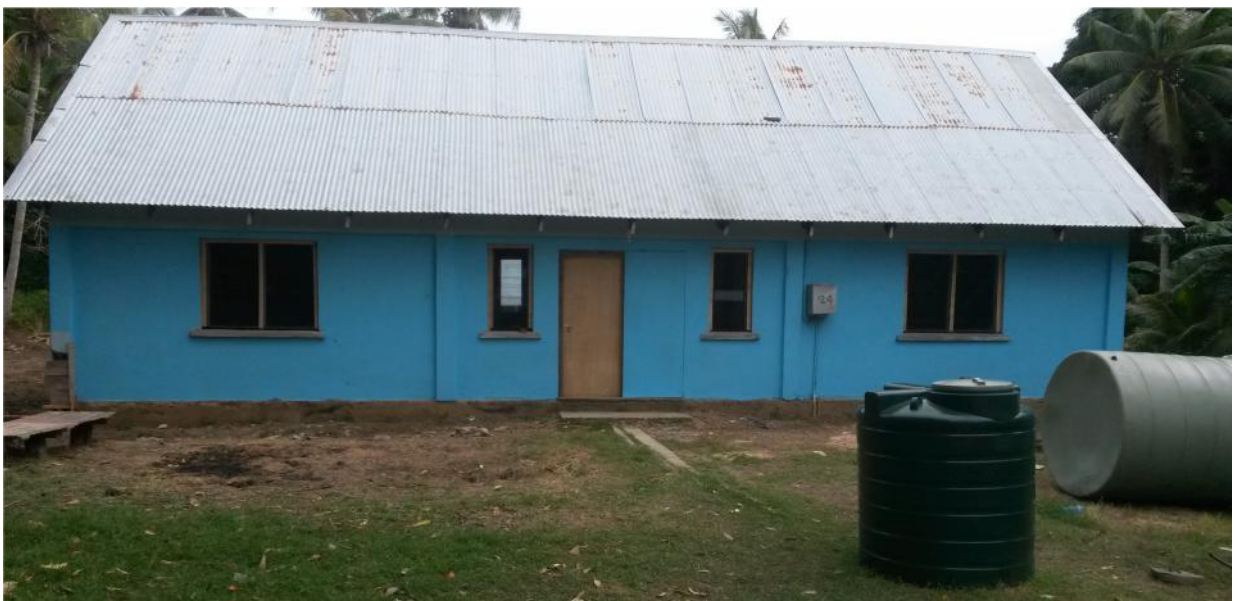
Figure 4: Building being renovated on Ono Island for geological office & accommodation.
